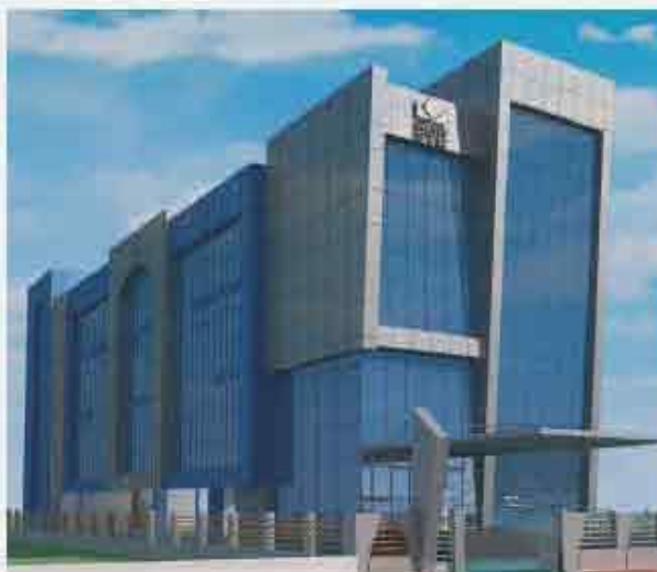
The new building of STC Chennai Branch is coming up at Guindy Industrial Estate, Chennai.
